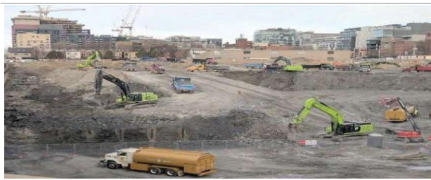
Figure 1.5: Exemplar Excavation Site [1]
