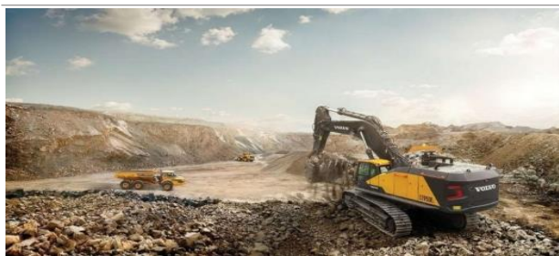
Figure 1.6: Exemplar Construction Site [2]
